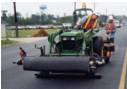
IMAGE K: Mechanical placement of the GlasGrid System.
