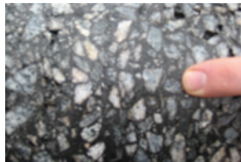
IMAGE C: GlasGrid remains intact after 20 million ESALs of traffic loading.
