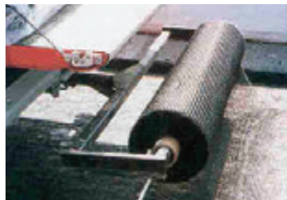
IMAGE L: Manual placement of the GlasGrid System.
