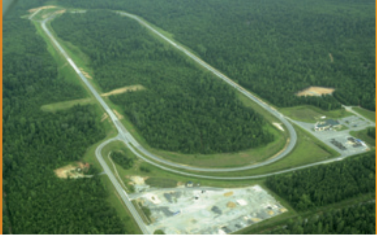
IMAGE B: GlasGrid was installed at the National Center for Asphalt Technology (NCAT) pavement test track in Opelika, AL.
